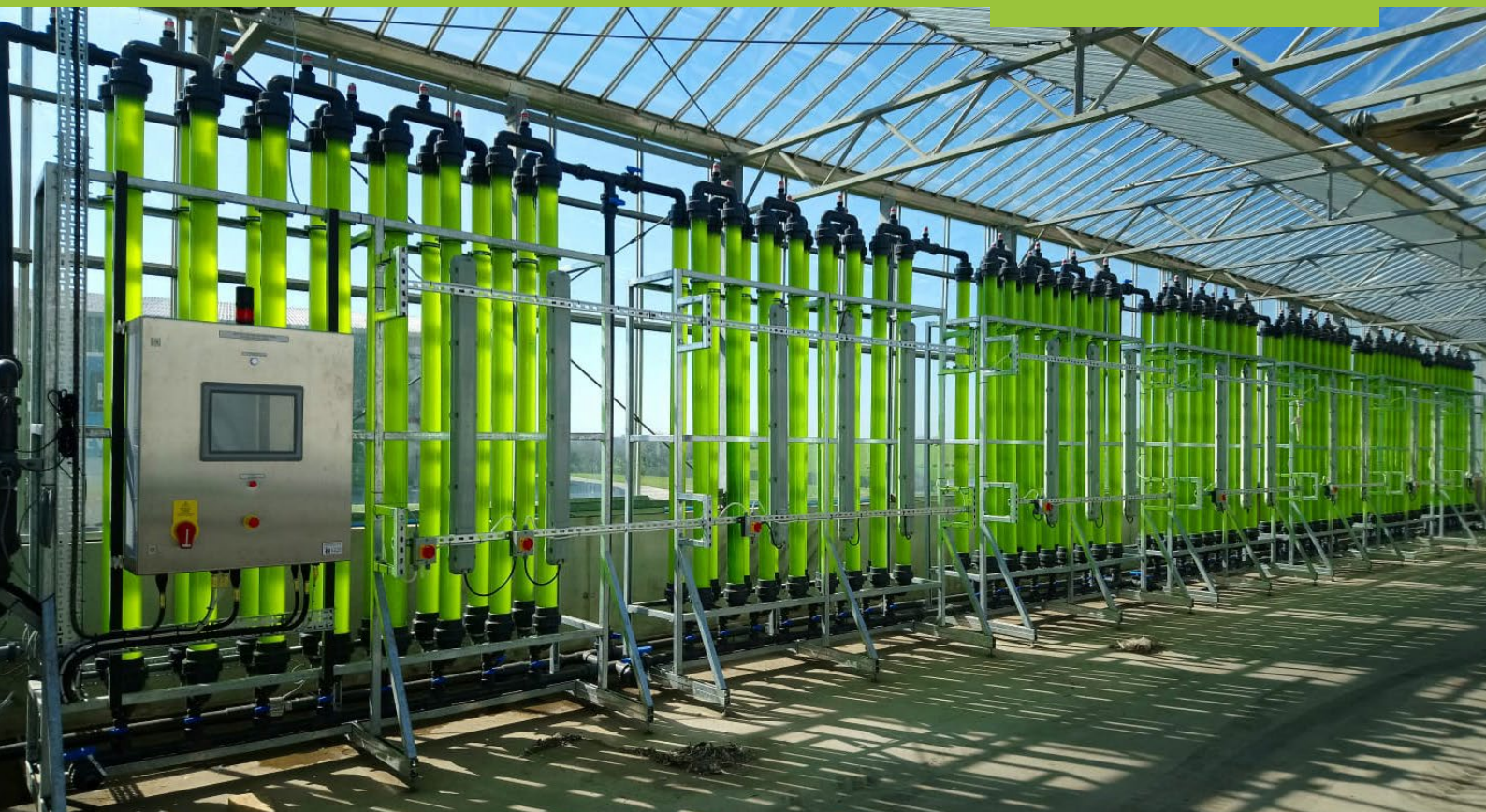
Reactor installation at Langage, Devon, UK
