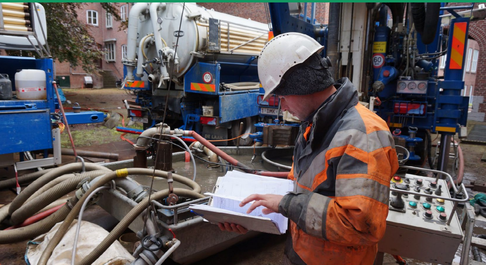
Test drilling at the Brunssum site of the D2Grids project
