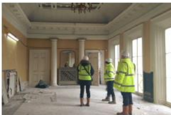
St Clements - John Denham Building
