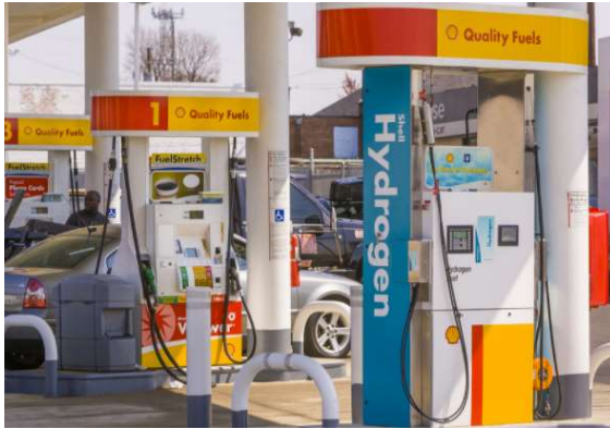
Figure 17: Hydrogen Dispensing at a Standard Forecourt 44
