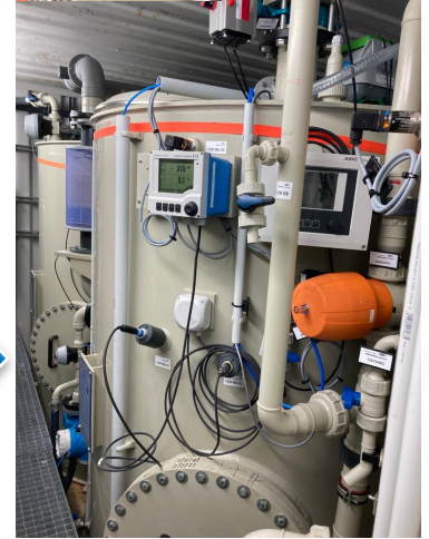
4 m 3 Reactor 1 (anoxic, lipid accumulation)
