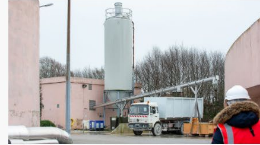
Saint-Omer WWTP, FR CAPSO
