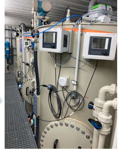
4 m 3 Reactor 2 (micro-aerobic, biomass growth)
