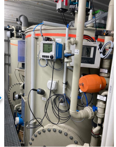
4 m 3 Reactor 1 (anoxic, lipid accumulation)
