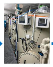
4 m<sup>3</sup> Reactor 2 (micro-aerobic, biomass growth)
