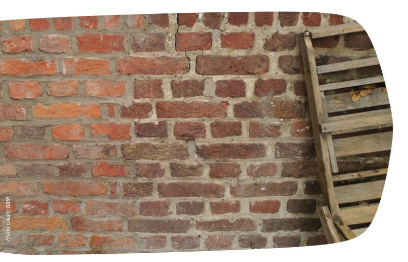
Given the different colours of the bricks present, as well as the differences in mortar, it seems wise to divide up these bricks into separate batches from the time of dismantling onwards.
