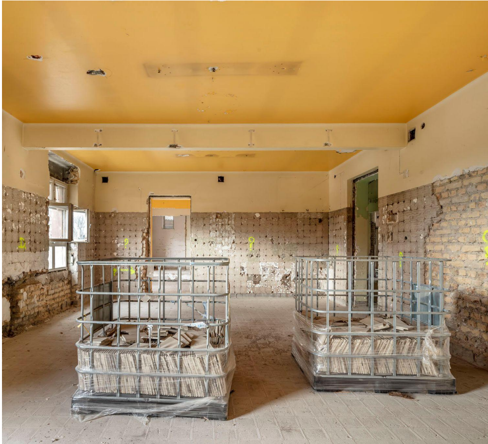
Dismantled tiles, packed for transport © Luc Boegly
