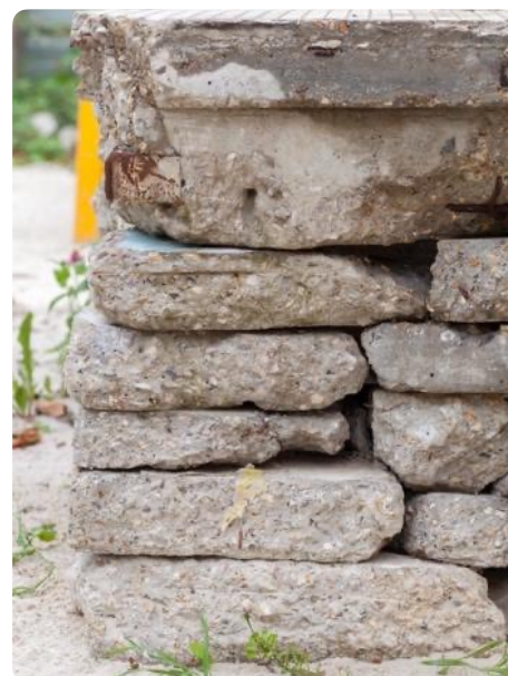
Landscape masonry in concrete rubble resulting from the demolition of a housing building built between 1966 and 1970. The Clos factory is a demonstration site of the potential for reusing concrete elements resulting from demolition. It was fitted out and built from materials resulting from the demolition of buildings as part of the Clos-Saint-Lazare urban renewal project.
