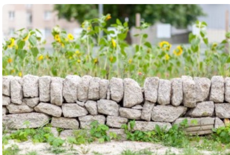
Landscape masonry in concrete rubble resulting from the demolition of a housing building built between 1966 and 1970. The Clos factory is a demonstration site of the potential for reusing concrete elements resulting from demolition. It was fitted out and built from materials resulting from the demolition of buildings as part of the Clos-Saint-Lazare urban renewal project.
