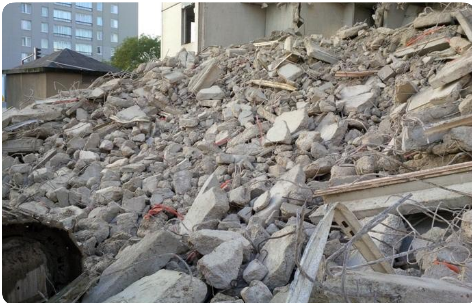
Concrete rubble deposit from the demolition of a tower at Clos Saint Lazare in Stains (FR).
