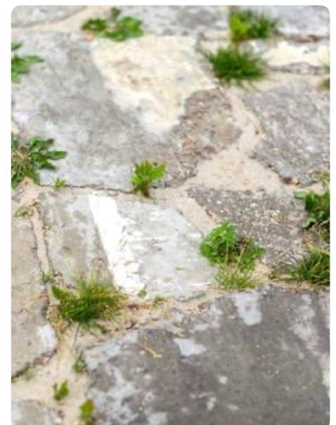
The "Opus uncertum" of Clos Saint Lazare in Stains (FR), 2017. The concrete resulting from the demolition of a residential building built in 1959 was reused on site to cover the ground of the outdoor spaces.
