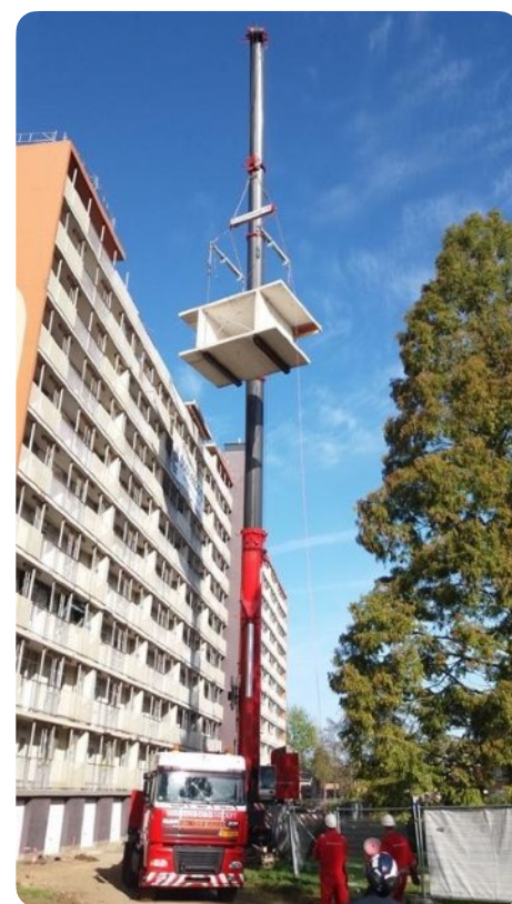
Super Local Project. This experimental project carried out in 2017 in the Netherlands implemented a reclaim process of three-dimensional concrete modules extracted from an old housing building, for the construction of individual houses. The modules consist of slabs and walls, which were sawn before being crane-mounted and transported by truck to the nearby reclaim site. Client: HEEMWonen. Architect: SeC Architects. Contractor: Jongen Construction. Research unit: Zuyd University of Applied Sciences, Research group SURD.
