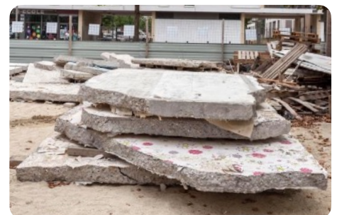
Example of a concrete wall after nibbling removal © Alexis Leclercq
