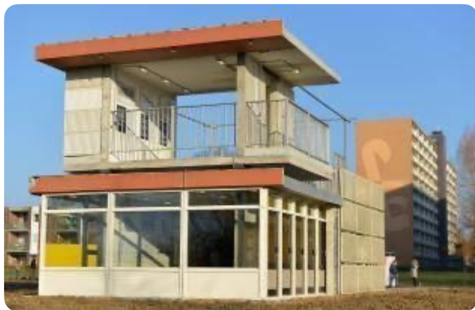
Super Local Project. This experimental project carried out in 2017 in the Netherlands implemented a reclaim process of three-dimensional concrete modules extracted from an old housing building, for the construction of individual houses. The modules consist of slabs and walls, which were sawn before being crane-mounted and transported by truck to the nearby reclaim site. Client: HEEMWonen. Architect: SeC Architects. Contractor: Jongen Construction. Research unit: Zuyd University of Applied Sciences, Research group SURD.
