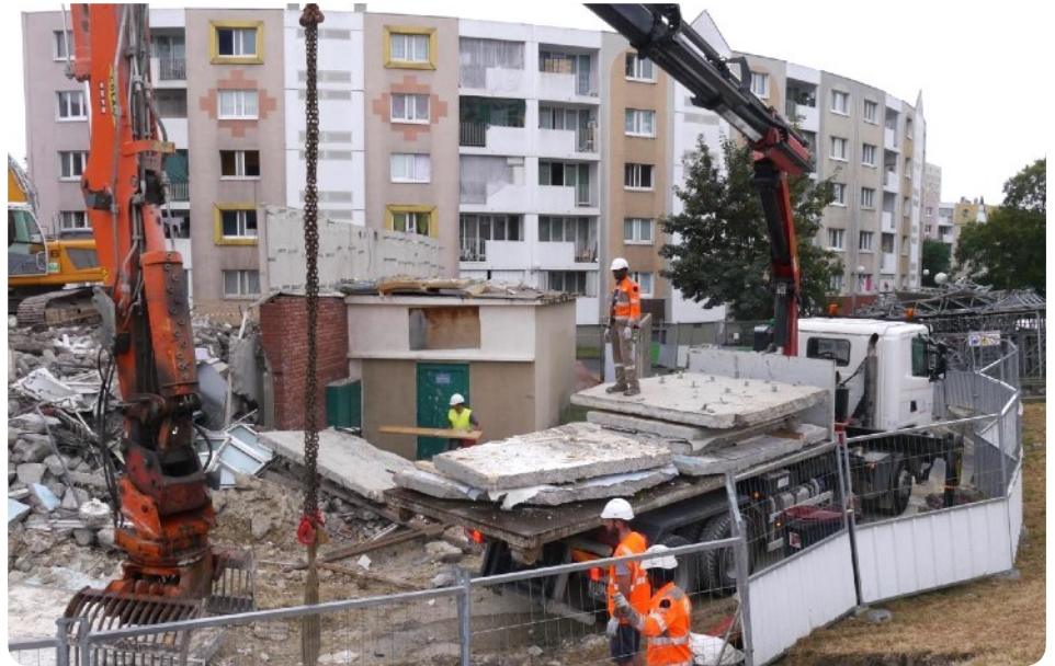
Transport of concrete elements
