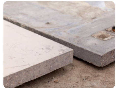
Sawing of concrete walls before re-use © Alexis Leclercq
