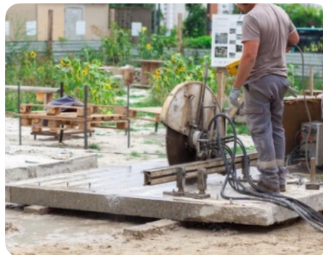
Sawing of concrete walls before re-use © Alexis Leclercq
