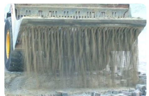
Removing pavers using a riddle bucket © VSB Sierbestrating
