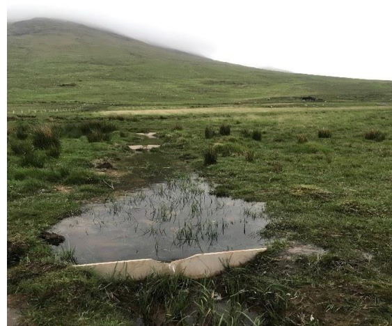
Timber weirs blocking drainage in Bundorrhaga site
