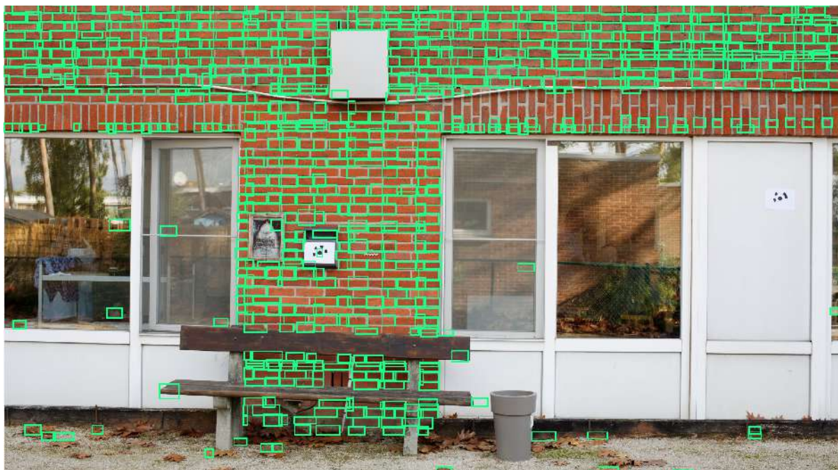
Figure 2. Result after initial training, showing detection of horizontal bricks while vertical bricks are left undetected (source BBRI).
