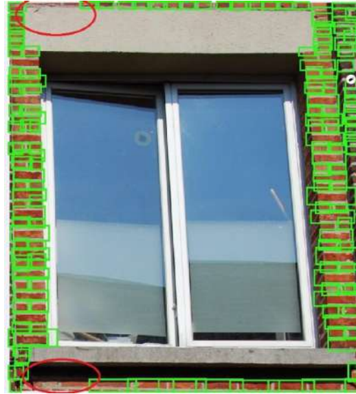
Figure 3. Red ellipses indicate areas where brick detection failed due to partial brick visibility.
