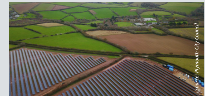
Photovoltaic installation Creacombe Solar, UK.
