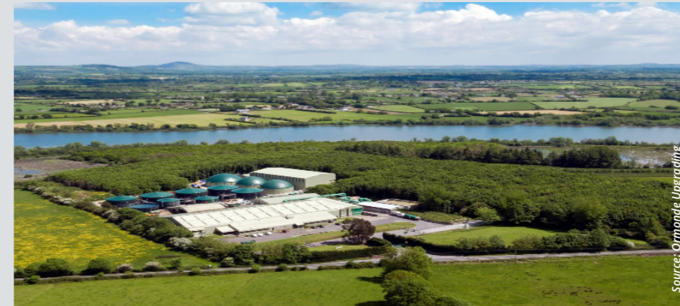
A view over the Ormonde Upgrading biogas and biomethane production site in Waterford, Ireland.
