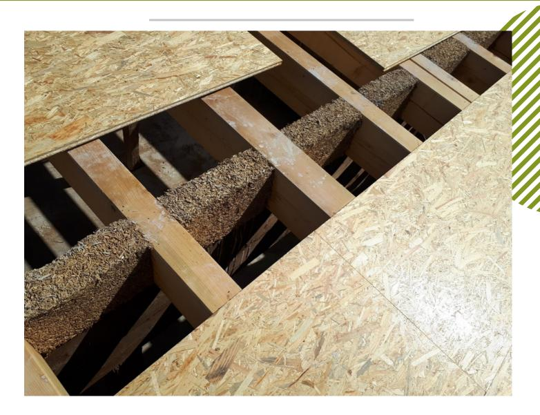
For the platform itself we used standard OSB panels, which are strong enough due to the small gaps they need to traverse and comparatively cheaper than any other solution like multilayer boards. Since the material is not waterproof and is constantly under atmospheric influences, they needed to be sealed off properly. Here, bituminous sheeting was used which was welded in rolls onto the boards.
