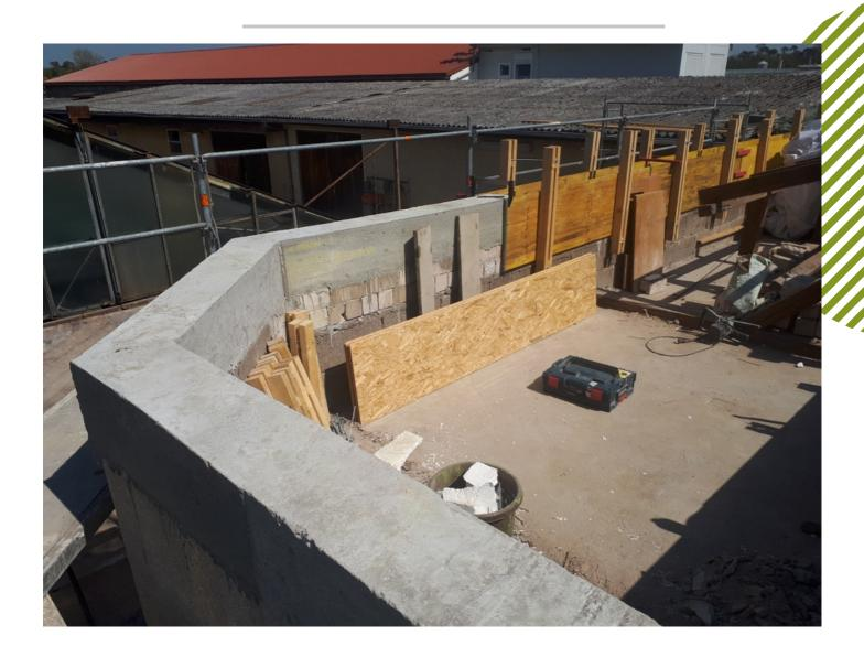
The next step in the construction of the platform involved the placement of the large wooden support beams, which were laid out in a pattern so that the later installed greenhouse post could be placed exactly on top. This reduced the amount of total material necessary since the main load on the platform results from the greenhouse itself and not the growing systems or the live load.
