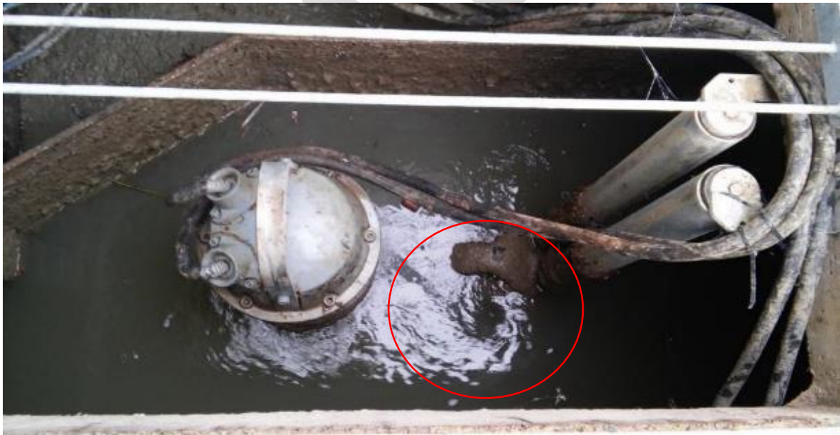
Figure 10 – Surface Vortices on Pump 2
