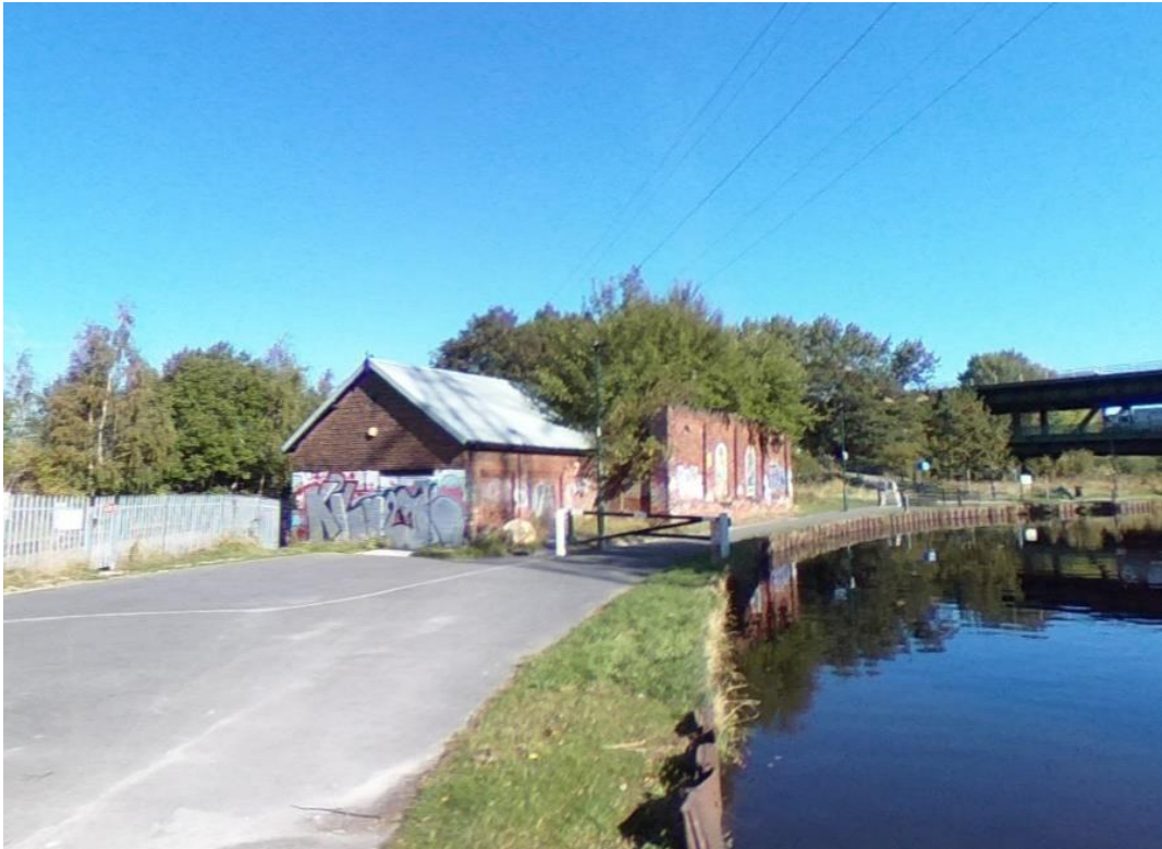
Figure 3 – Tinsley Pump Station building
