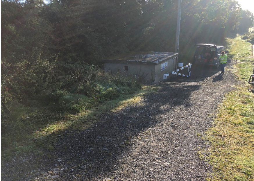
Figure no. 16: Lock 16 on the Grand Canal PS (viewed from Digby Bridge)
