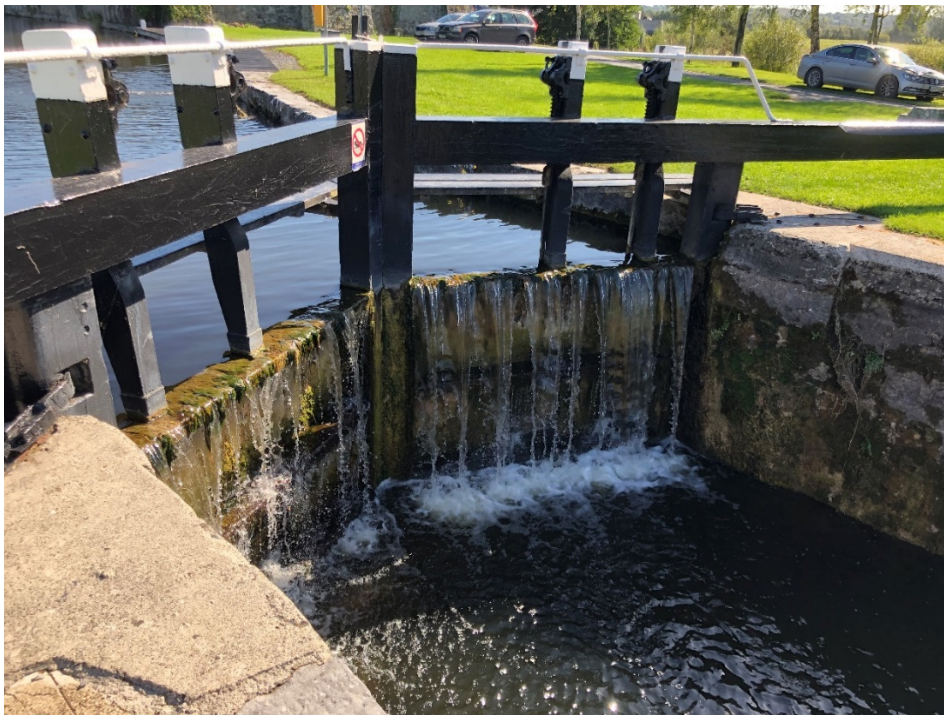
Figure no. 31: Flow overtopping lock gate at Lock 35
