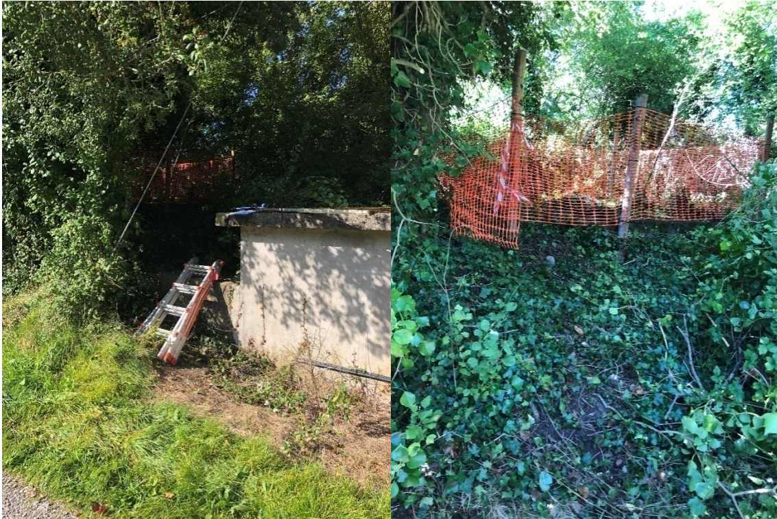
Figure no. 21: Lock 18 PS Outfall – located behind pumping station
