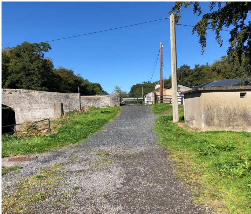
Figure no. 17: Lock 17 on the Grand Canal PS (viewed from Digby Bridge)
