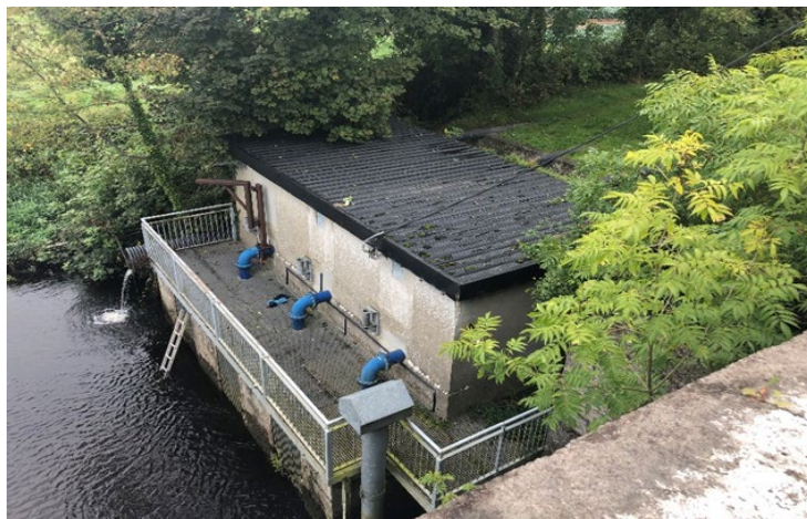
Figure no. 14: Leinster Aqueduct PS (viewed from Grand Canal)
