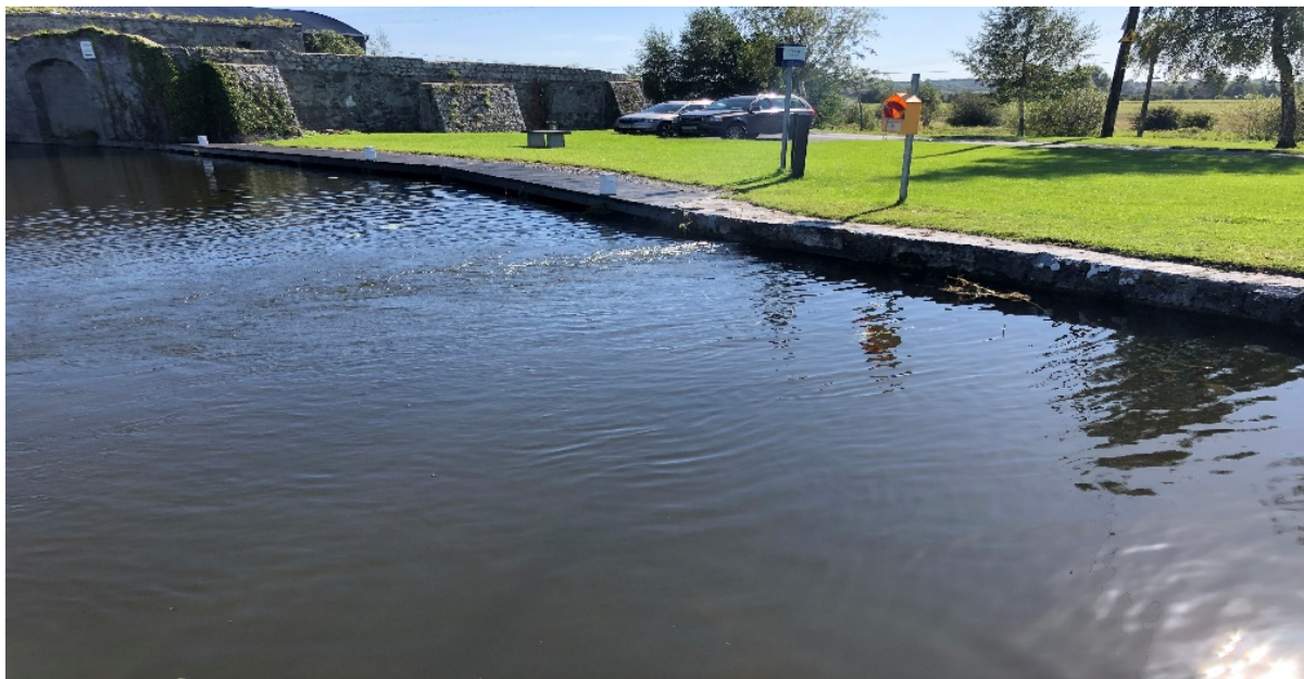
Figure no. 28: Lock 35 PS Outfall
