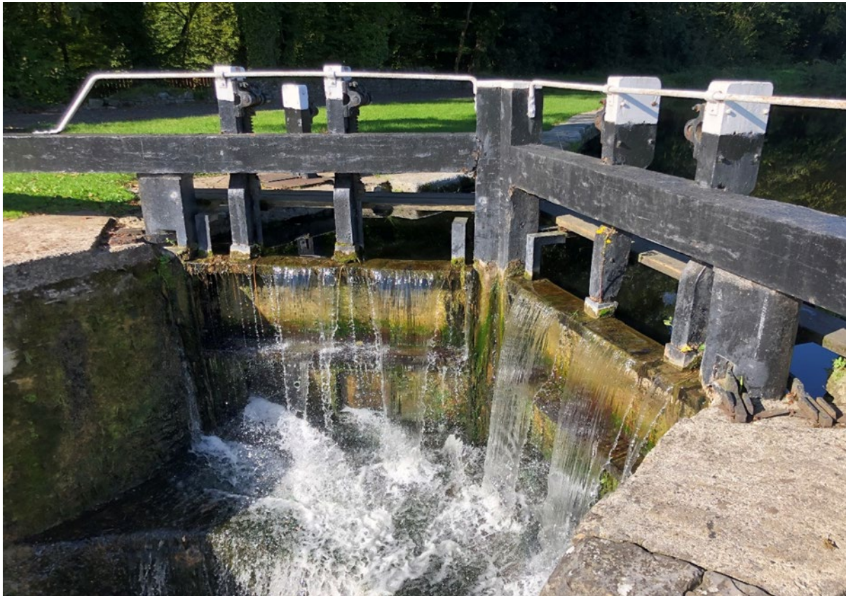
Figure no. 25: Over topping of lock gate at Lock 17
