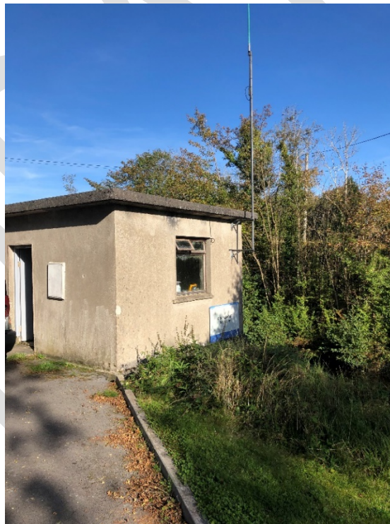
Figure 1- Drumleague Pump Station
