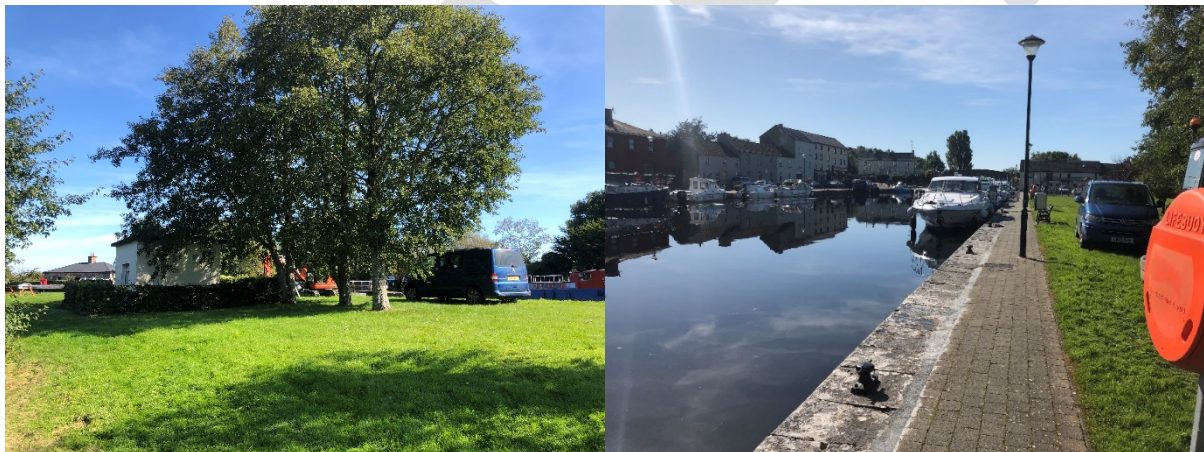
Figure 1 – Richmond Harbour PS ( Left); Richmond Harbour Outfall (right)
