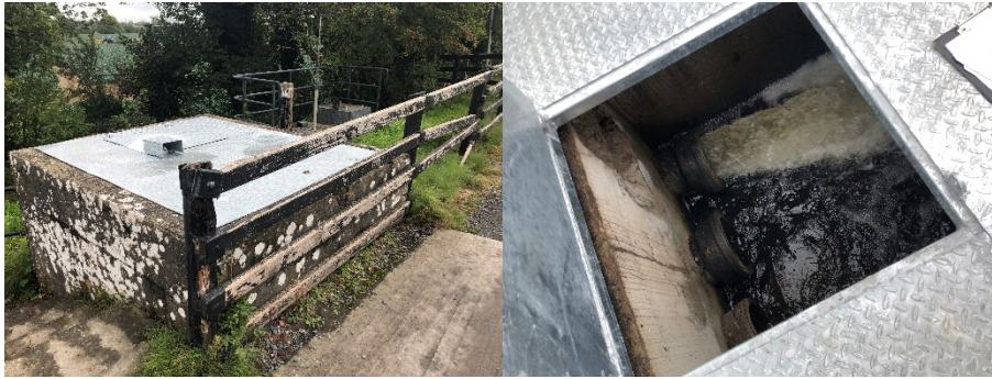
Figure 2 -Leinster Pump Station Outfall
