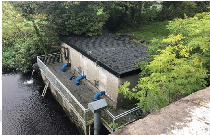
Figure 1- Leinster Pump Station (viewed from Grand Canal)
