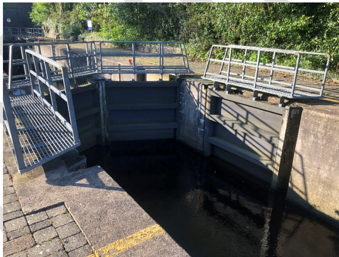
Figure 1- Drumshanbo Dual Lock Station
