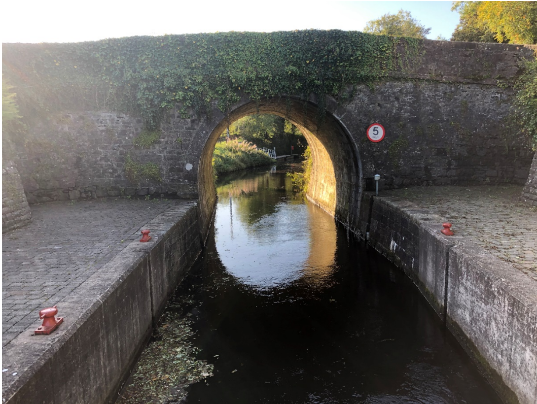
Figure 3 -Drumshanbo PS – Outfall
