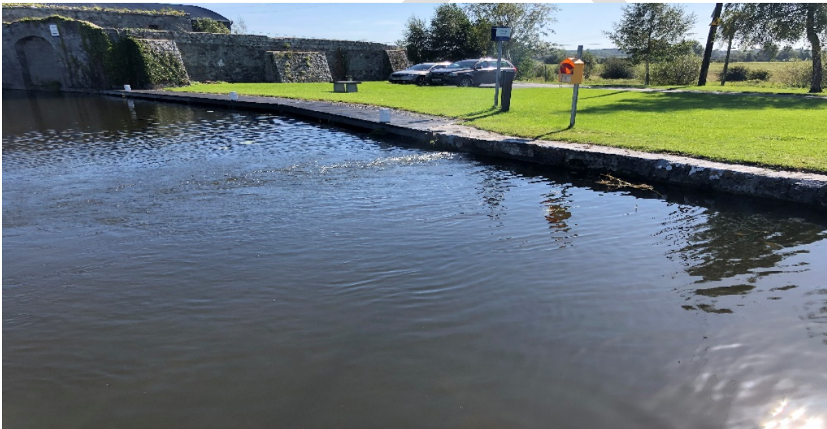
Figure 6 Lock 35 PS Outfall
