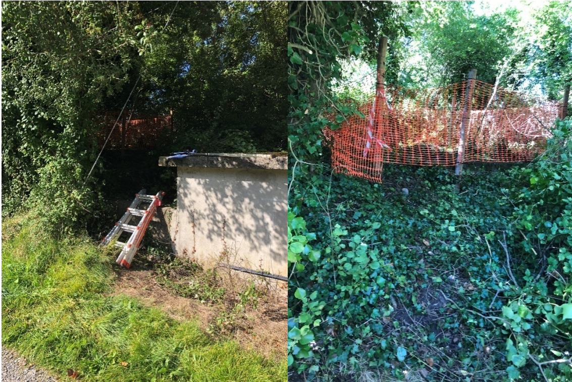
Figure 10 Lock 18 PS Outfall – located behind pumping station
