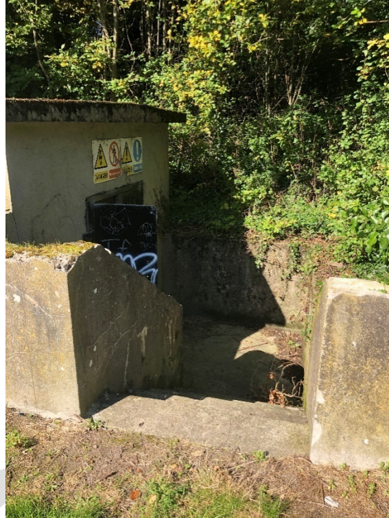
Figure 9 - Lock 18 on the Grand Canal PS (viewed from Canal Path)
