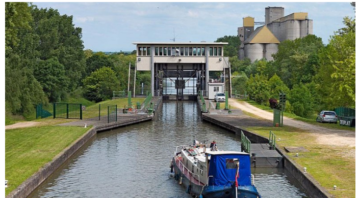
Figure 3 : Crissey pumping station
