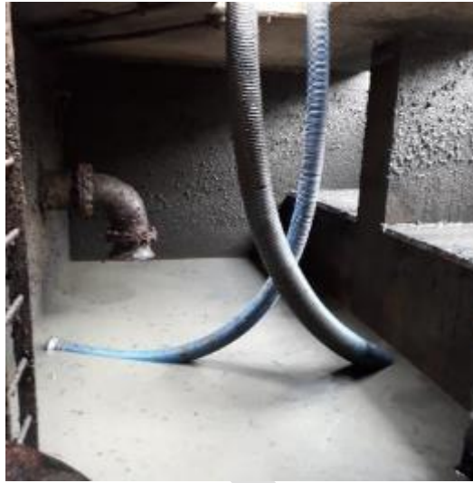
Figure 11 – Photos during Caen Hill wet well cleaning – August 2019
