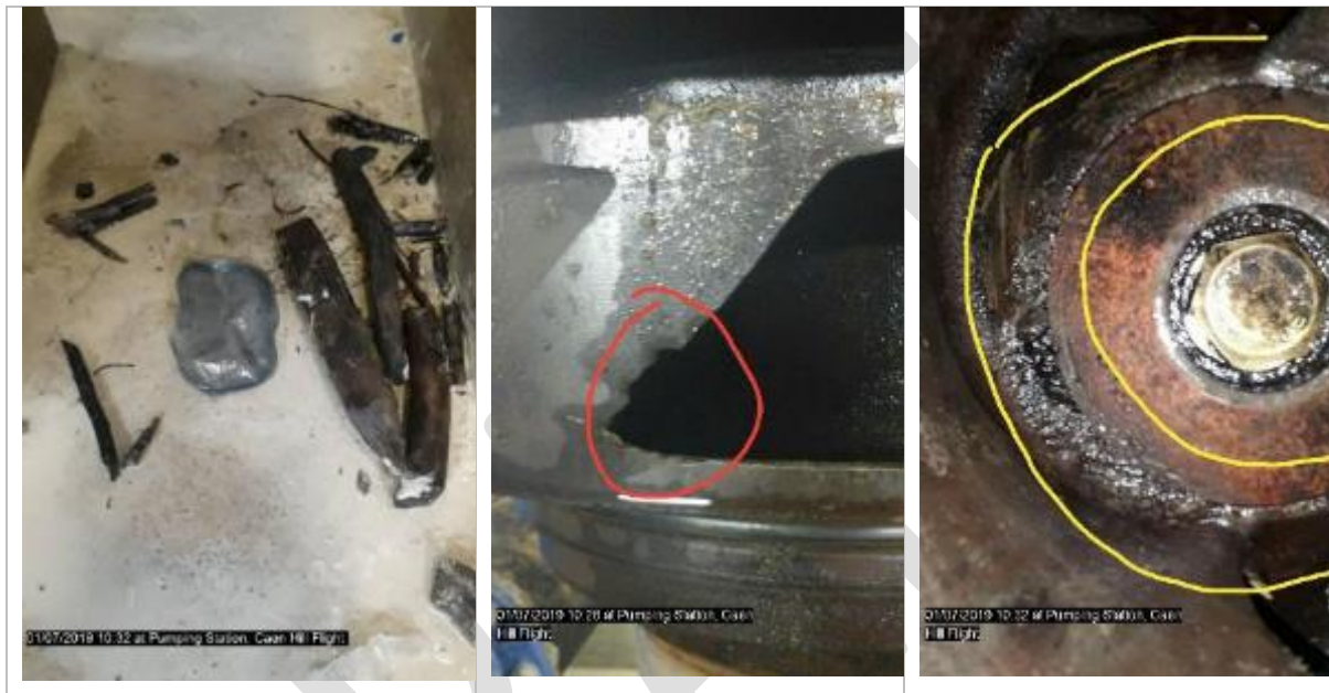
Figure 10 – Photos following Pump No.2 Inspection – July 2019
