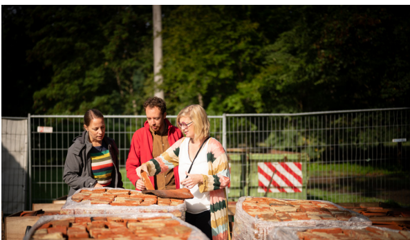
60 m 3 of hand-formed bricks are kept separately on-site to be reused later in the new construction.
