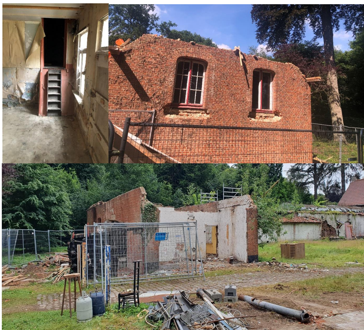
Picture 15: Ongoing deconstruction works of the southern, most valuable barn
