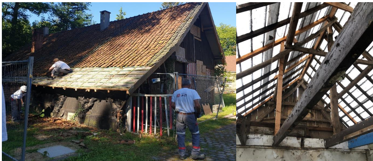
Picture 10: Dismantling of the roofs
