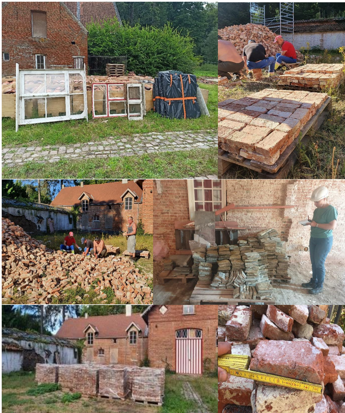
Picture 16: Cleaning, measuring and storing of the materials to be reused
