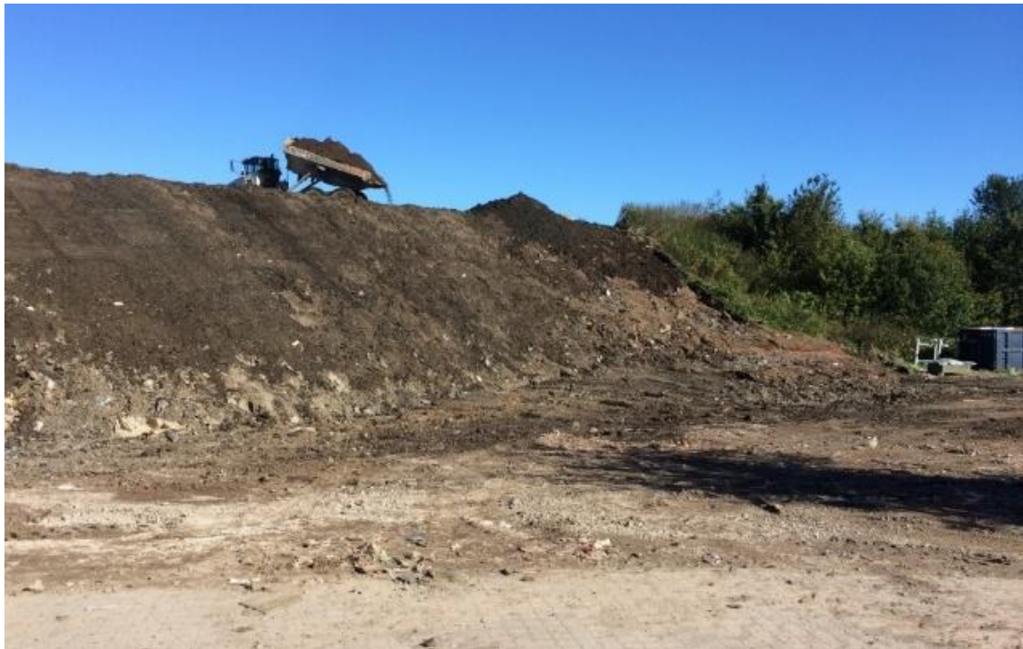
Figure 12-12 Site during the rehabilitation operations.
