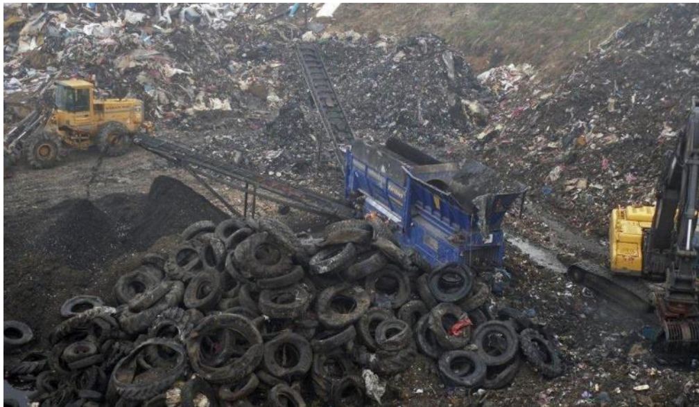
Figure 12-9 Landfill mining operations at Gerringe Landfill.
