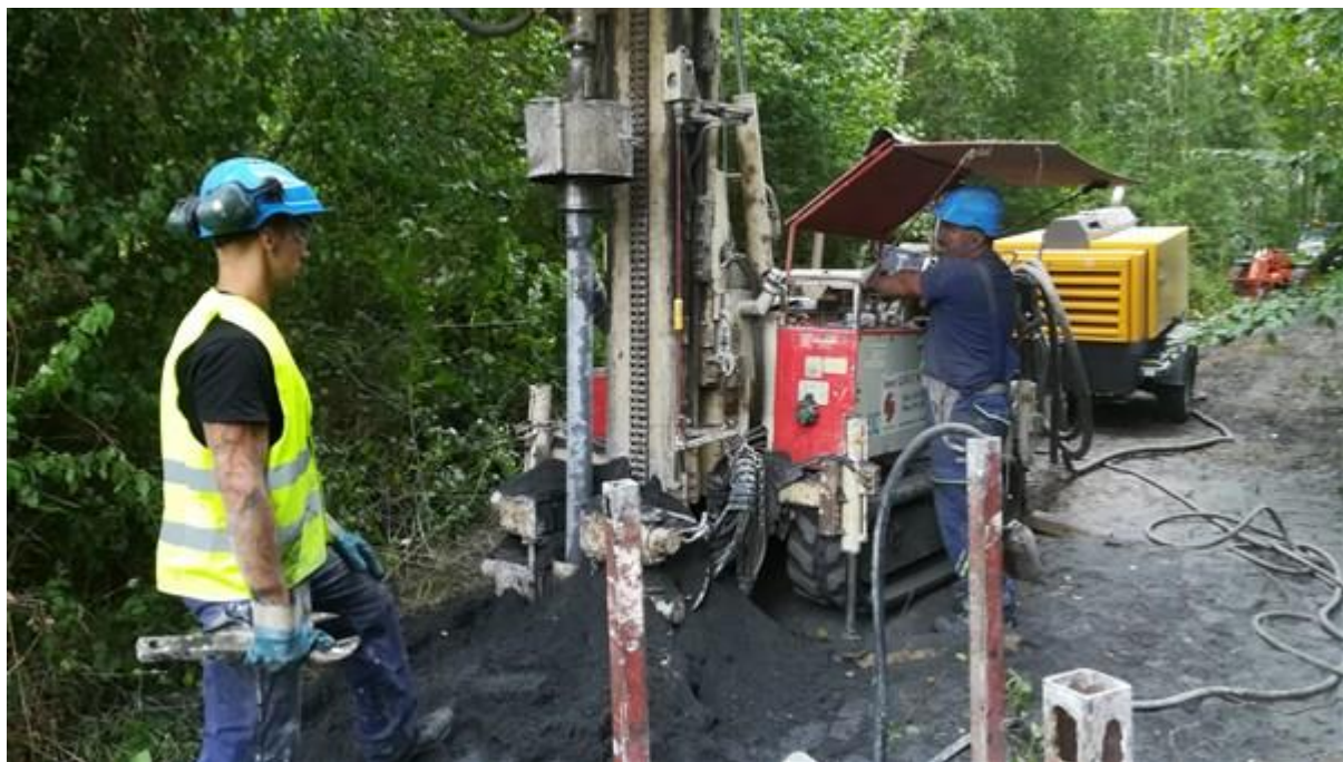
Figure 5-1 Down-the-hole hammer drilling in the fly ash deposits of the Onoz industrial landfill, one of the RAWFILL pilot site (Credit Photo: Atrasol).
