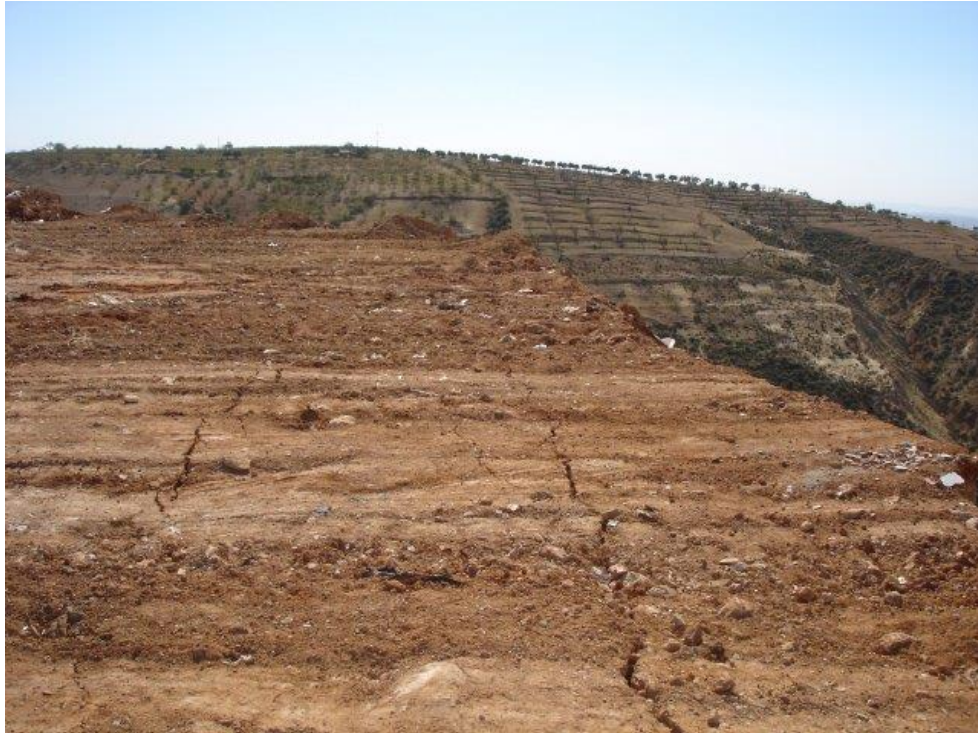
Figure 8-2 Horizontal cracks at the top of a landfill attesting stability problem (Credit Photo: Atrasol).
