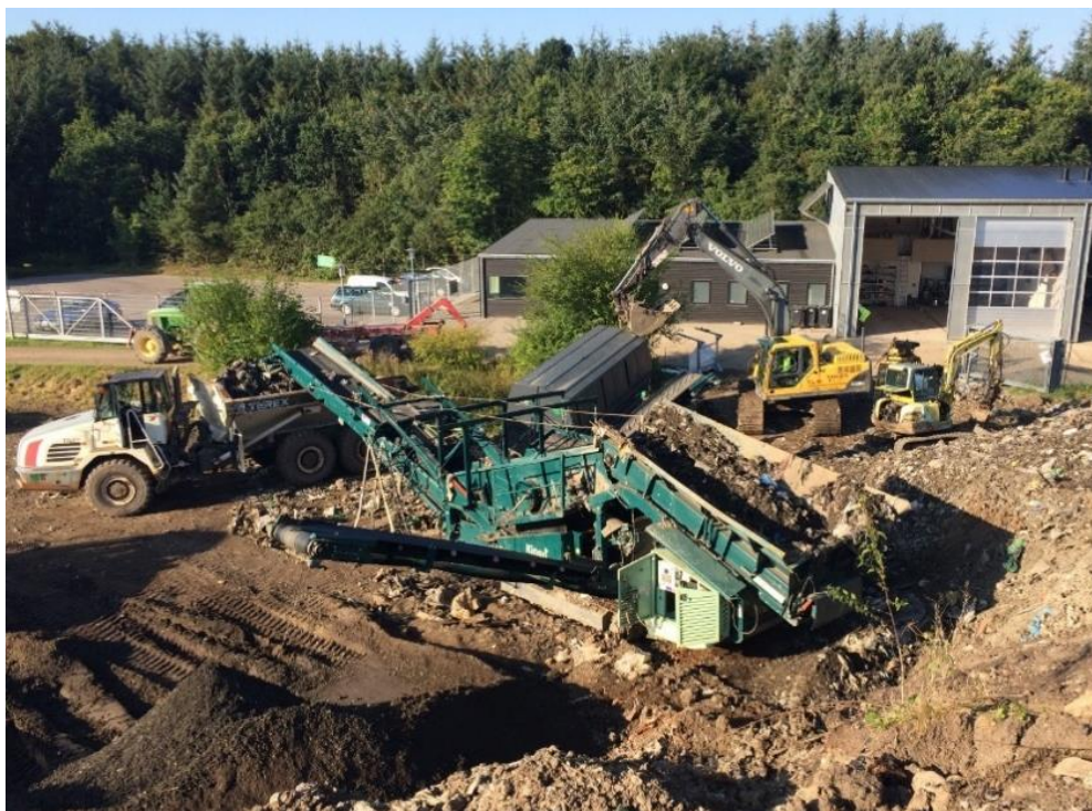
Figure 12-11 Landfill mining operations at Skårup Landfill.
