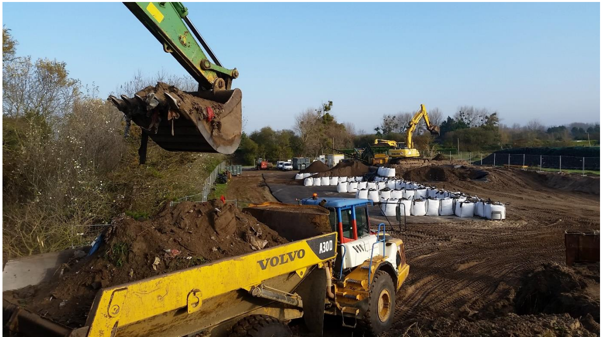
Figure 12-5 Landfill mining operations on la Samaritaine landfill. On the back, the sorting platform which is located next to the site. The asphalted area was used to store the fine fractions while waiting for the results of the geochemical analyses.
