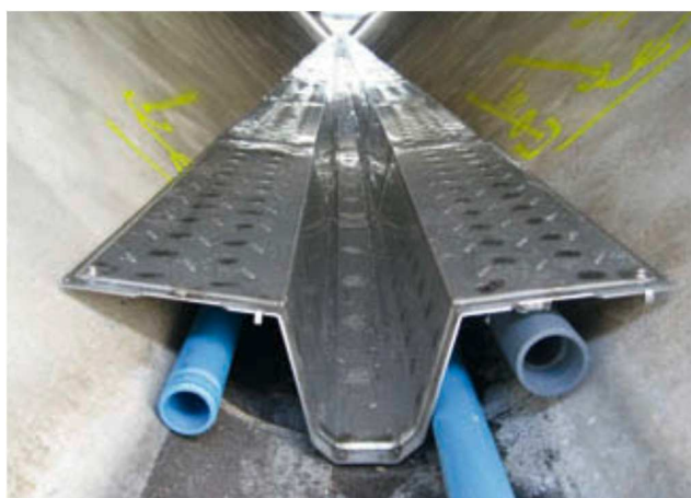
Figure 3-4: Heat exchanger elements during installation (Butz and Müller, 2010)
