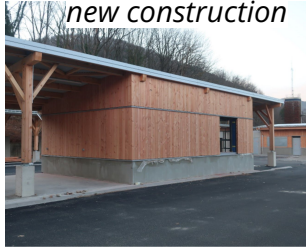
Kaysersberg waste collection centre (F), 7.535 m 2
