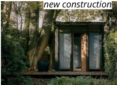
new construction Tree House (NL), 24 m 2
