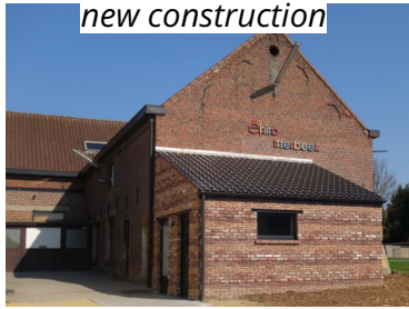
new construction Sanitary block (B), 18 m 2
