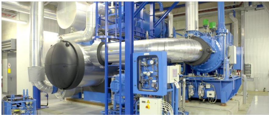
Figure 18. a. Friotherm Unitop 50 at Canavese district heating plant. [23] b. Friotherm Unitop 50 scheme [13]
