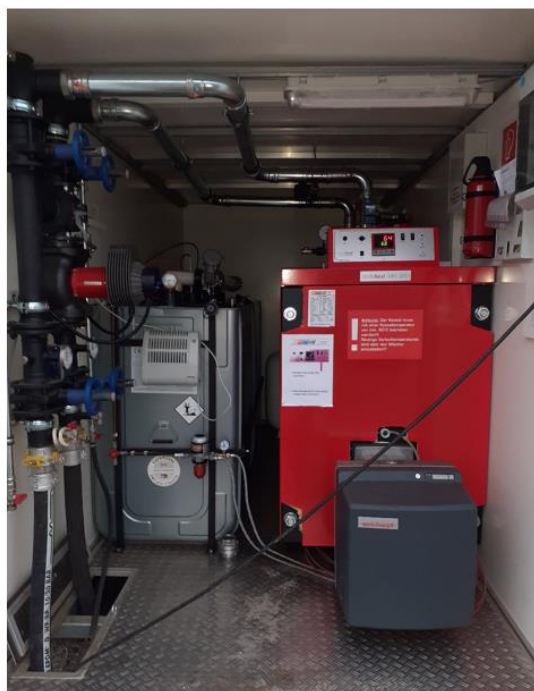
FIGURE 6. Installation for heat injection tests into the mine
