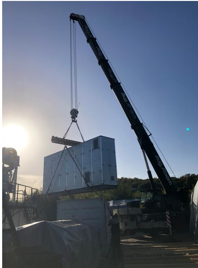
Figure 5. Delivery operations of the heat pump units
