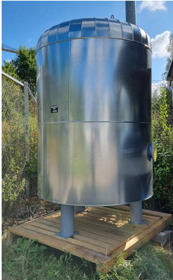
Figure 4. Buffer tank
