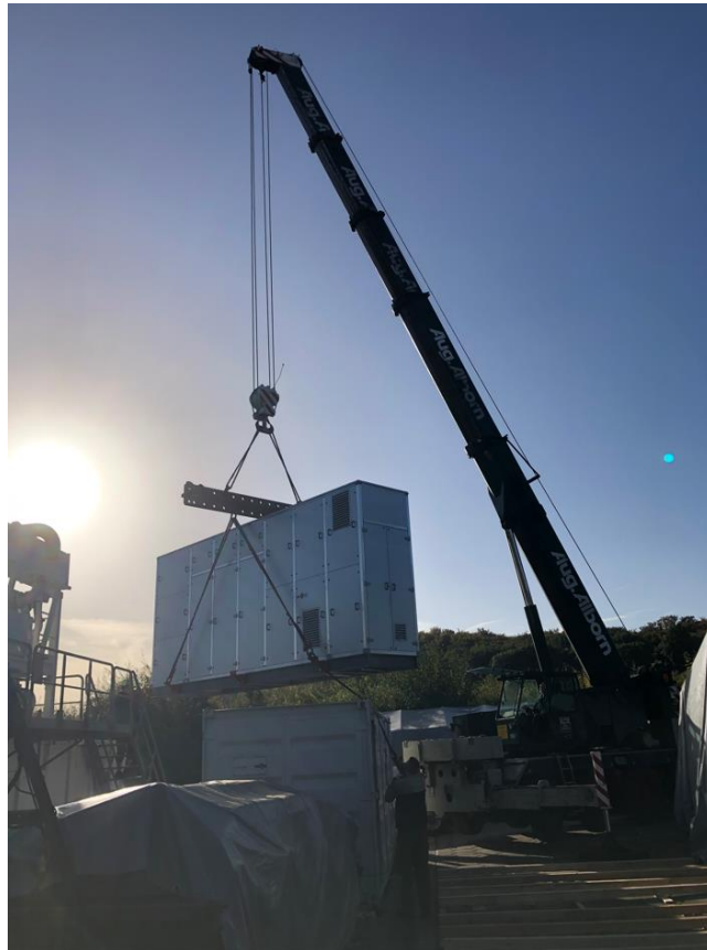
Figure 5. Delivery operations of the heat pump units
