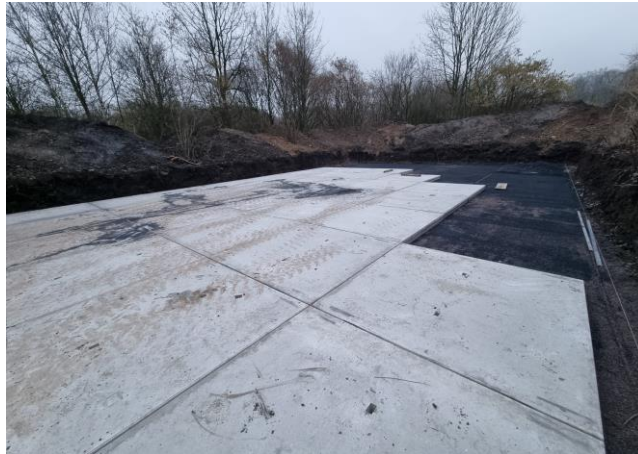
Figure 9. Construction of the foundation
