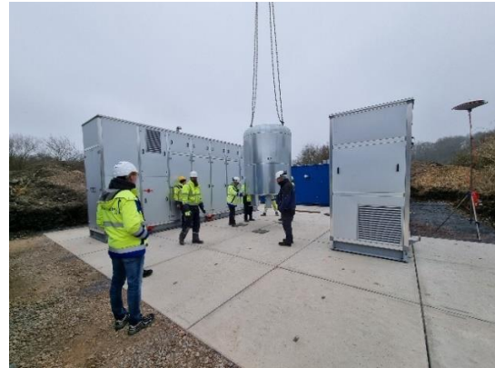
Figure 11.b. Final positioning of components
