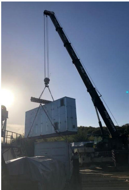
Figure 8.a. Delivery of the units
