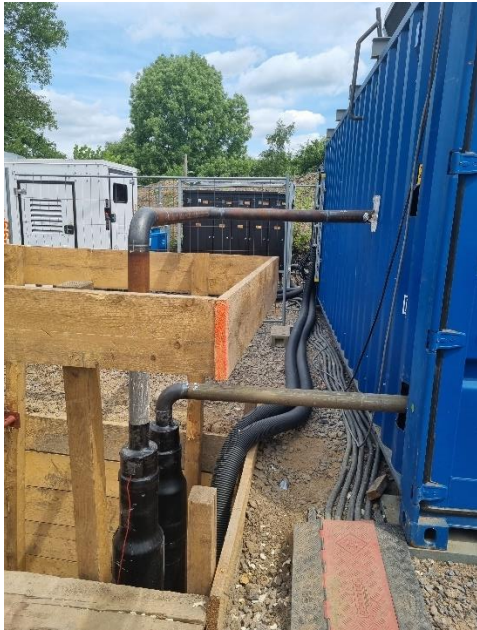
Figure 15.a. District heating connection
