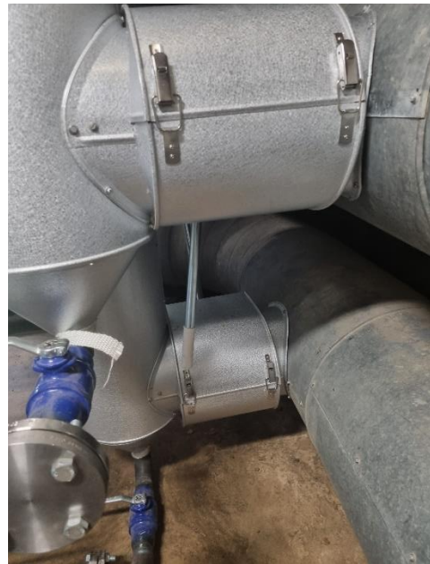
Figure 165.b. Connection to main DH pipes
