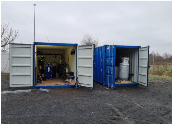
Figure 11.a. Construction work in containers
