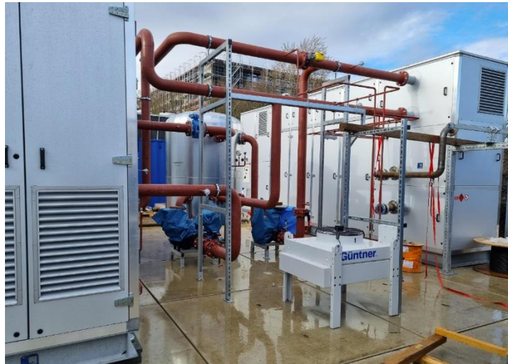
Figure 13. Hydraulic connection between the units
