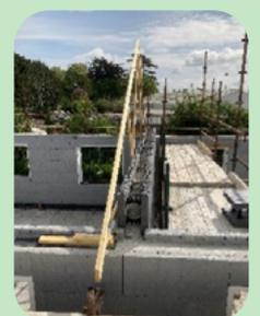
Figure 26: External ICF wall, part wall, and roof truss
