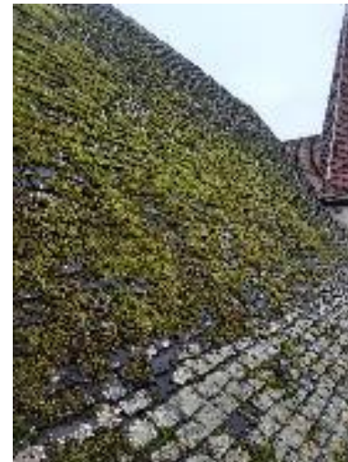
Moss on the roofs of poorly-maintained historical buildings Source: TMH ( https://vigipatrimoine.fr/entretien )
