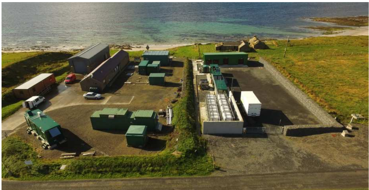
Figure 6: EMEC site and sea access
