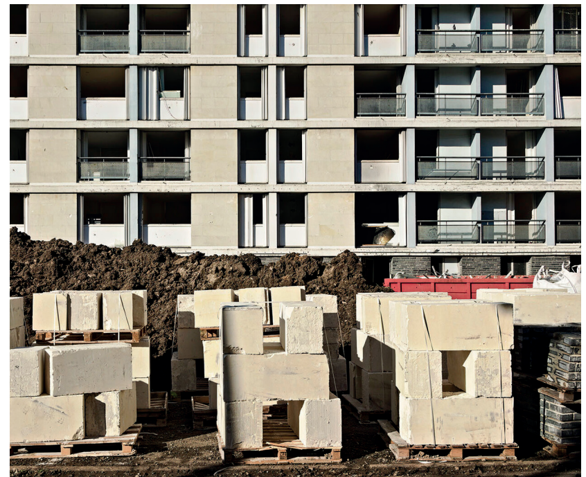
Reuse of 360 cubic metres of self-supporting solid tufa stone facades on a site in Tours FR . © F.Paillet - Tours Habitat
