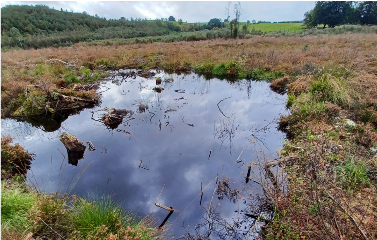
Figure 3.2: Completely flooded borrow pit, with the water approaching the top of the bund and flooding back up ditches and over the bog surface.
