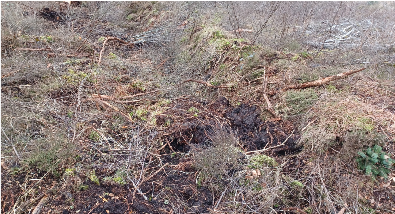
Figure 2.5: Detail of a completed section of bund, recovered with vegetation. The borrow pit is situated to the left of the bund and has been partially filled with brash and spare vegetation.
