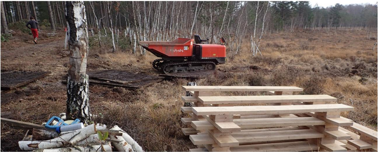
Figure 9. Walk-board constructed by Jura Natura Service.
