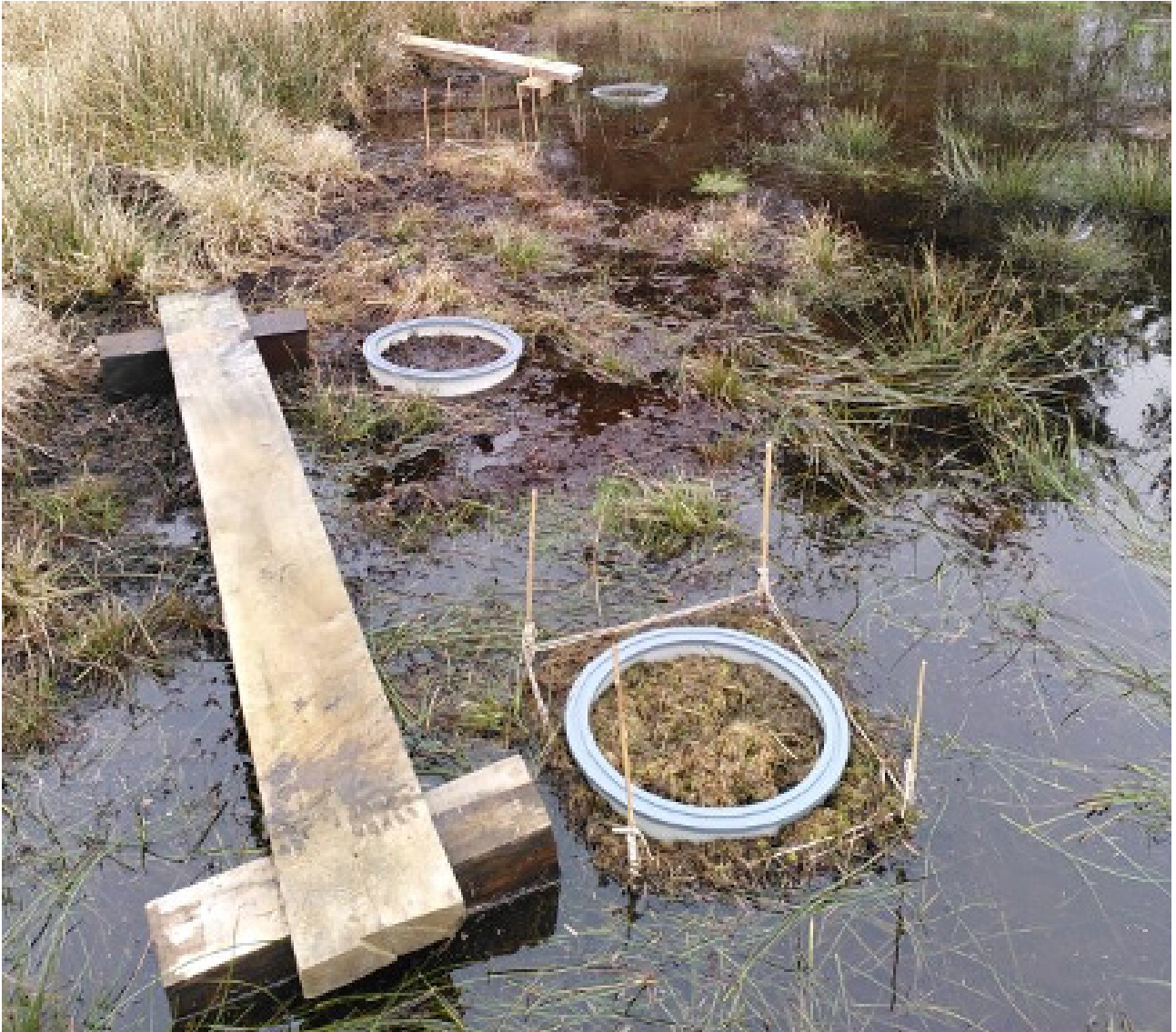
Figure 7: walk-board constructed by Jura the CD35 installed to have access to the collars to do fluxes measurements.
