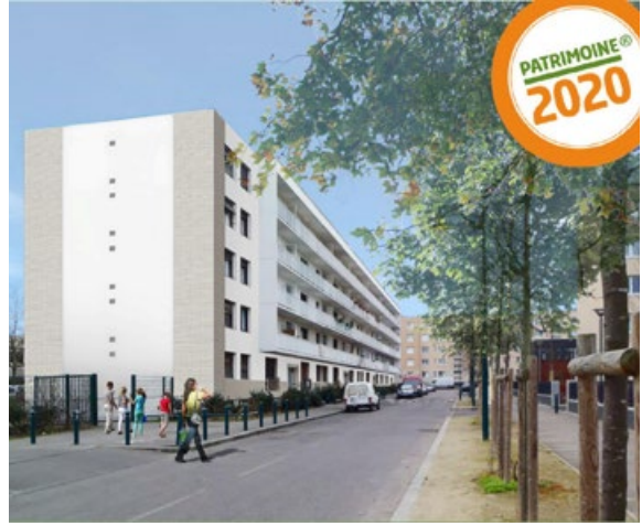
View of the building after renovation
