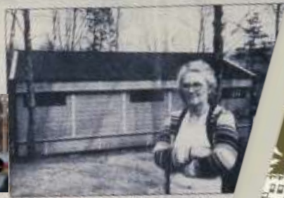
Constance Melnick stands in front of a newly completed, low-cost house.
