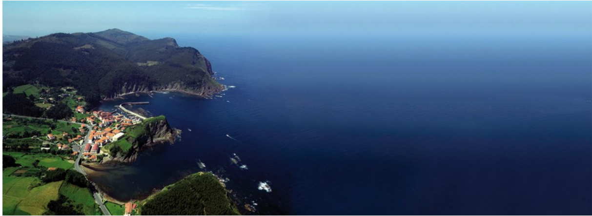
Figure 3-4 Overview of BiMEP site and facilities (from www.bimep.com )
