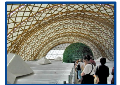
Modern timber techniques in the Japanese Pavilion at Hannover Expo (right).
