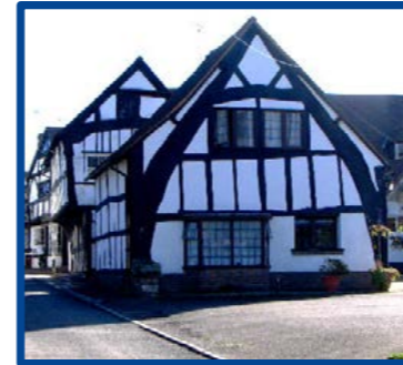
Traditional dowel-connected timber-framed building, England, (left). Photo credit: Doug Elliot
