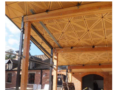
Images, (left to right): dowel connected EWP; schematic of assembly; double-curved EWP roof structure at Royal Holloway University, UK (image courtesy of Buckland Timber, UK)
