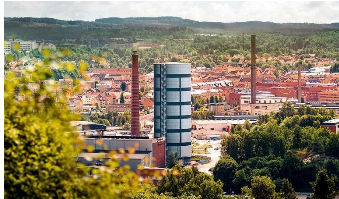
Figure 9: Borås thermal energy storage (source: Veolia)
