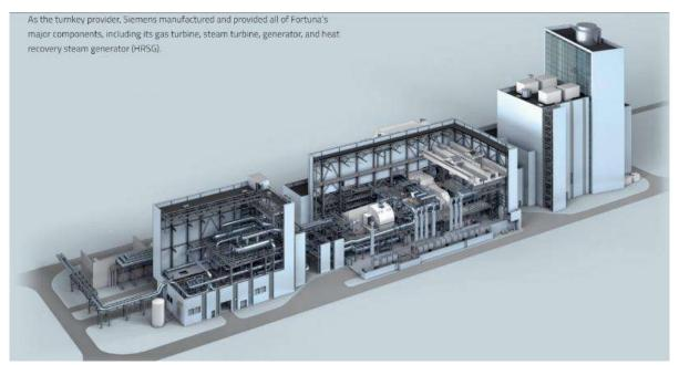
*Figure 35: Gas fired power plant in Dusseldorf making use of cogeneration.*
